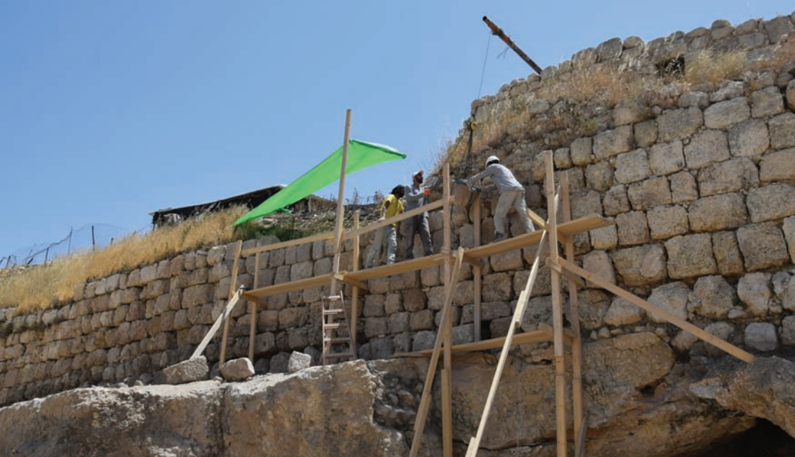
During the reconstruction and consolidation of the west wall of the Citadel.
