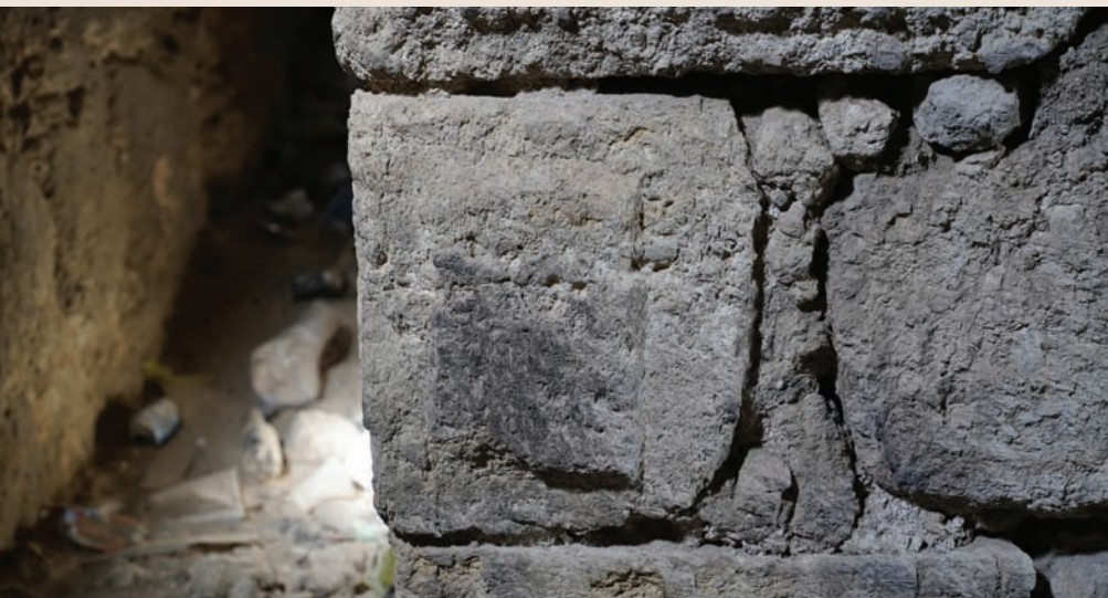
Embossed masonry in the lower part of Al-Burj Citadel's wall
