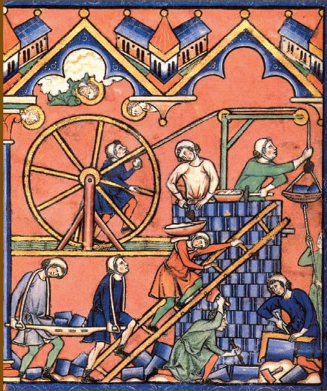
The use of a treadwheel crane and other devices in the building of a tower in a 13 th -century drawing
