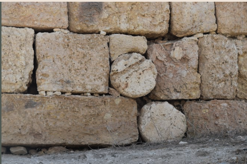
Detail of opus gallicum technique in the western wall of Al-Burj Citadel
