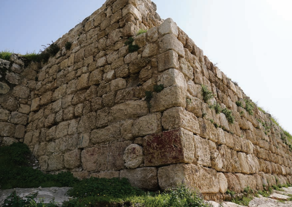
Opus gallicum technique in the north-west corner of Al-Burj Citadel
